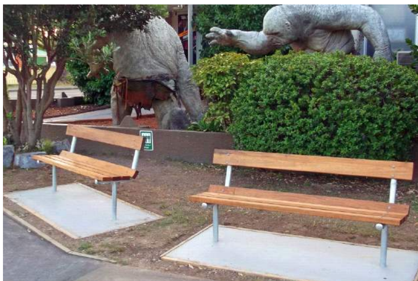
Newly-installed Longmarch Seats in Miramar, Wellington
